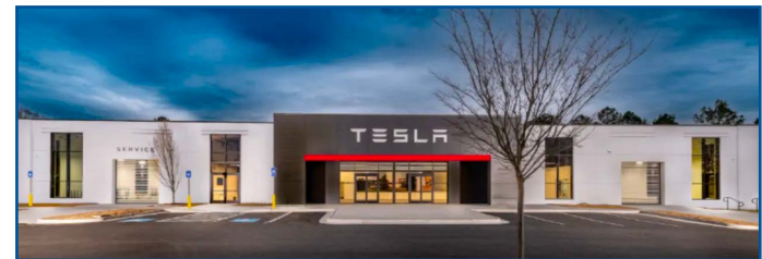
Tesla - Under Construction
